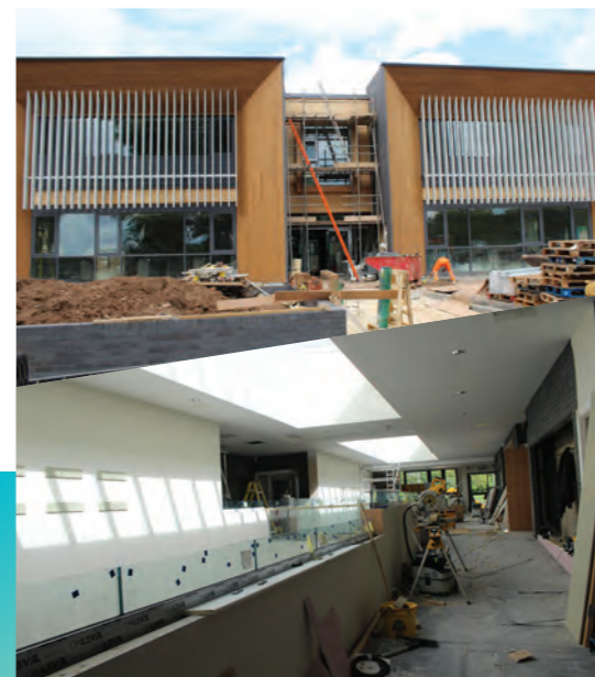
Internal work gathers pace and brise soleil installed
