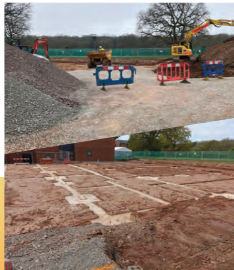
Earth works began
