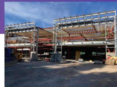
Steel work continues
