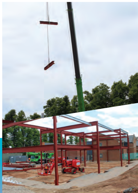
Steels craned in
