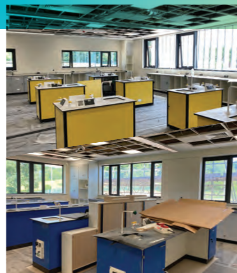
Internal labs fitting out under way
