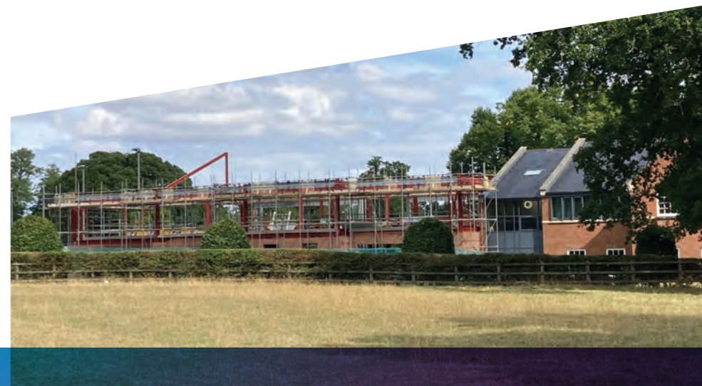
Work begins on brick work
