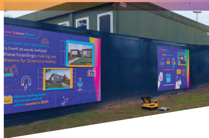
Site hoardings go up
